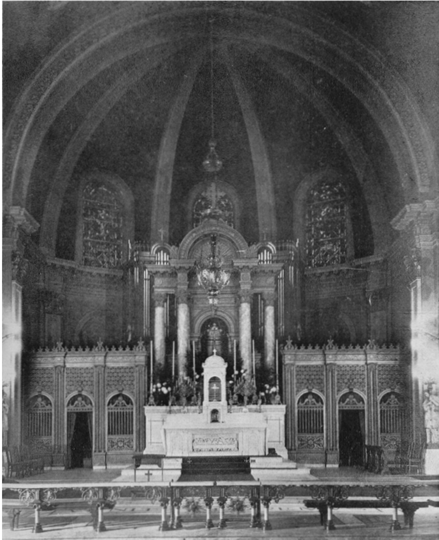
Figure 25 - Re-designed sanctuary, with choir screen, and Casavant organ showing behind reredos. 187
