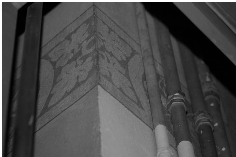
Figure 19 - Pre-existing stenciling in West Gallery, upper northwest corner.
