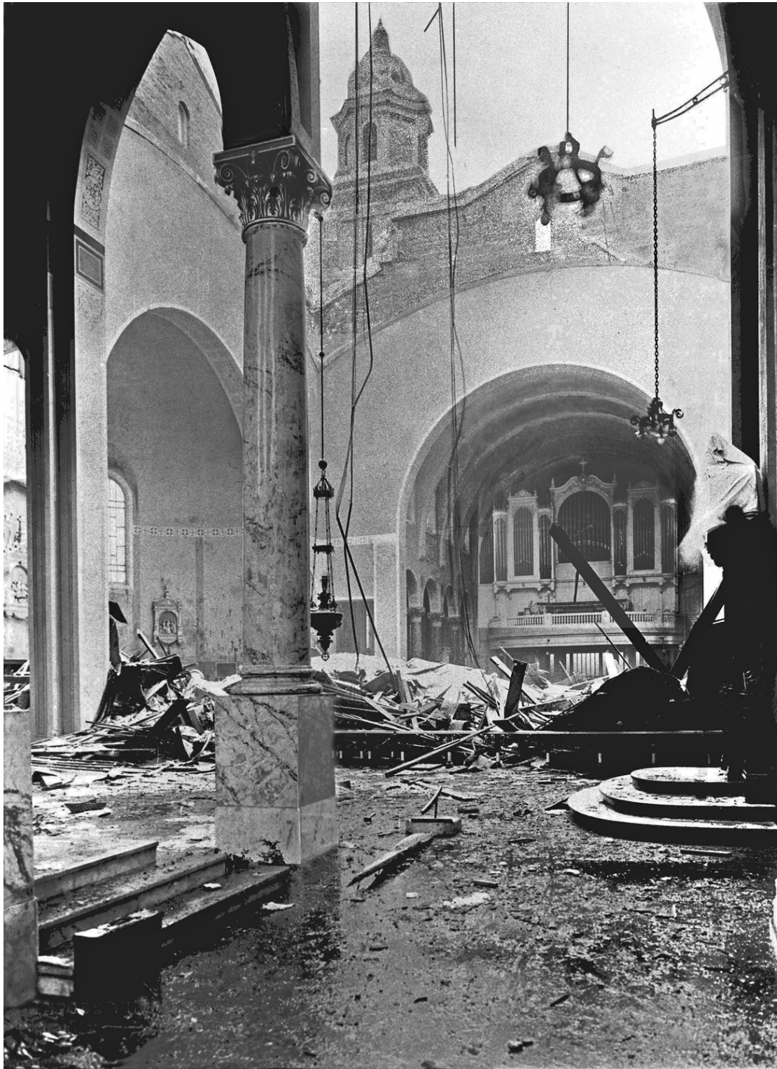
Figure 24 - Interior view looking west after the crash of the dome, 1916.
