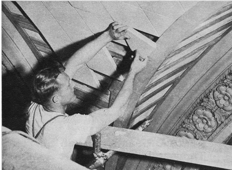
Accoustical Tile for Good Listening Goes on the Arches
