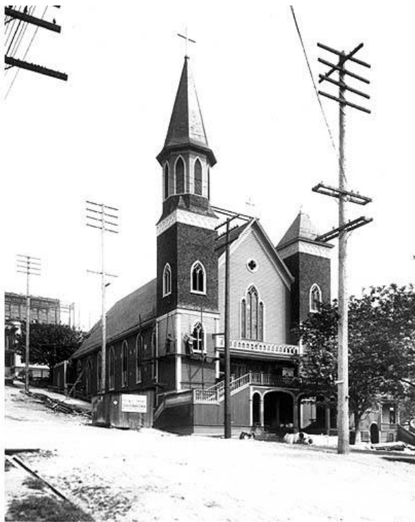
Figure 8 - Our Lady of Good Help rebuilt at Fifth and Jefferson. 38
