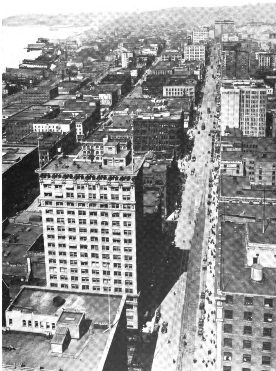
VIEW LOOKING NORTH FROM THE SMITH BUILDING, SECOND AVENUE
